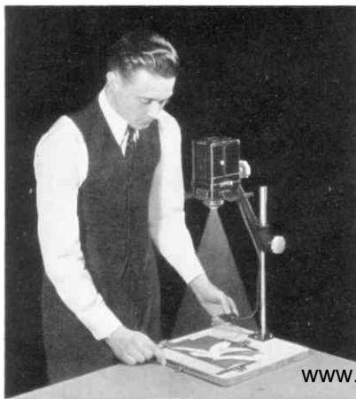
● Assembled, the Kodak Portable Miniature Enlarger makes brilliant enlargements from small negatives.
